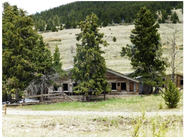
Figure 5. Alfred Bebee added additional rooms to his home as his family grew. The Bebee house is located next to the Vindicator Mine. Photo © by S. W. Veatch.
