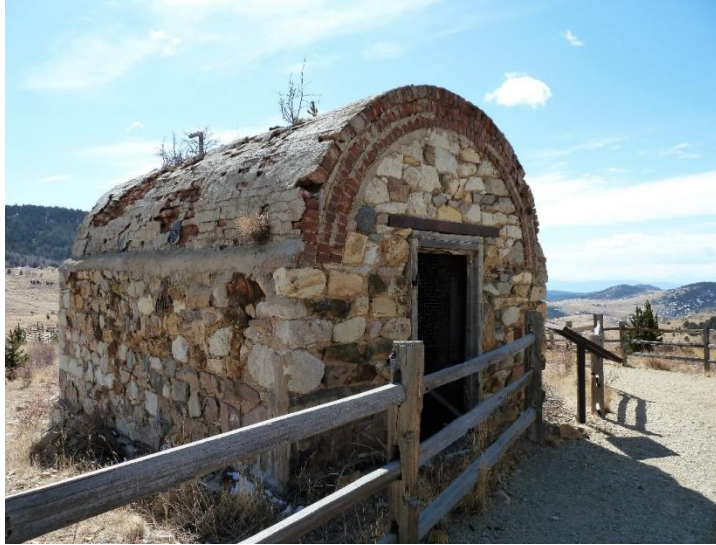
Figure 6. Dynamite storage building made of local rocks. The roof is made of bricks and is arched to allow an unwanted explosion's force to go through the roof, causing less damage, rather than the force going through the sides of the building, which would cause extensive damage. Photo © by S. W. Veatch.
